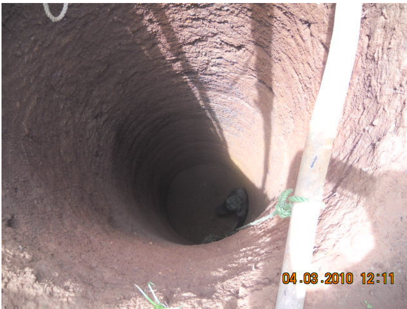
Well Under Construction- That's a worker at the bottom!
