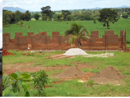
Form 3 Classrooms under Construction
